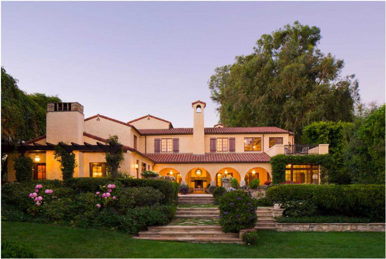
All of the touchstones of the Spanish Colonial architectural language are present in this Los Angeles home. Thick plaster walls, terra-cotta roof, rich stained-wood accents, and a shady, comfortable loggia all contribute to the Mediterranean character. (Photo: Manolo Langis)
